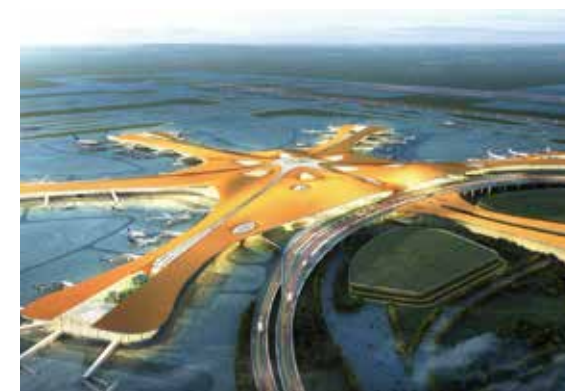
Daxing International Airport Project
