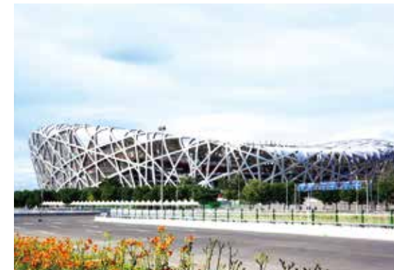
Bird's Nest Stadium Project in Beijing
